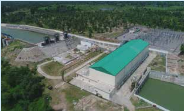
View of Dhukwan SHEP Power House building
