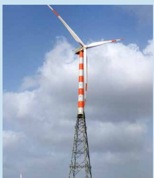
120 Mts High Hybrid Wind Tower at 63 MW WPP Distt. Devbhoomi Dwarka, Gujarat
