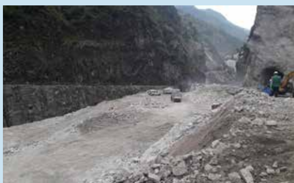
Dam excavation in progress at VPHEP
