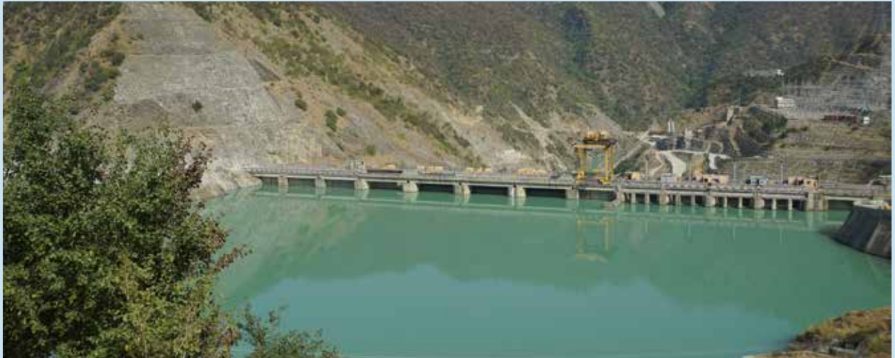
Upstream view of Koteswar HPP
