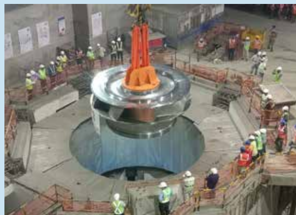
Erection of runner of first unit of Tehri PSP
