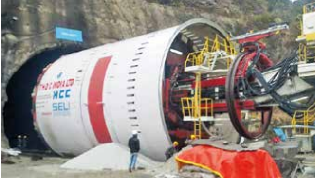
TBM pushing in progress at Vishnugad Pipalkoti (VPHEP) (4x111 MW)
