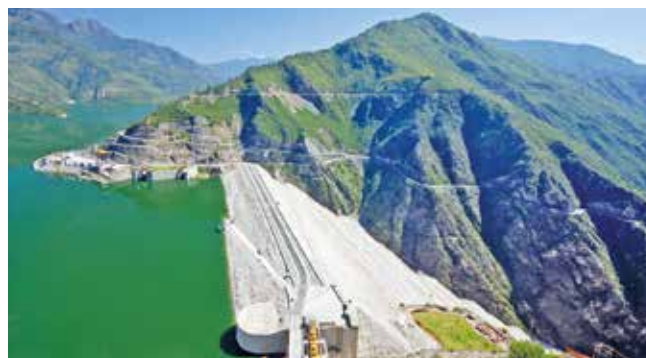
An overview of Tehri Dam & Reservoir
