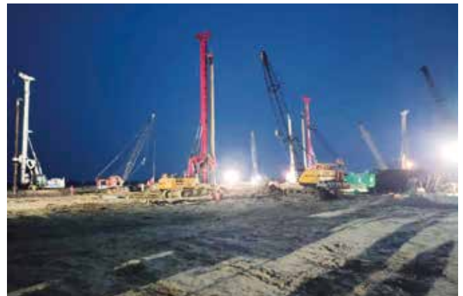
Job Piling work in progress at Khurja STPP (1320 MW)
