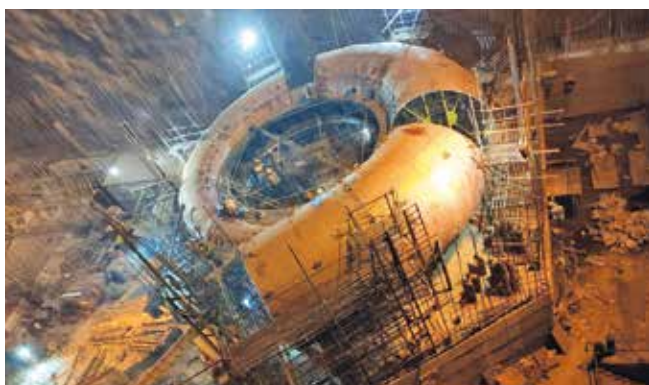
Unit-5 erection work is on progress at Tehri PSP (4X250 MW)
