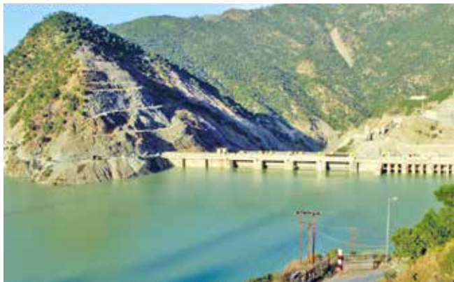
An upstream view of Koteswar Dam & Reservoir
