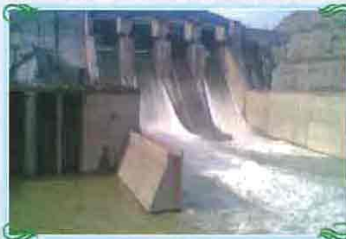
Down Stream view of Koteshwar Dam
