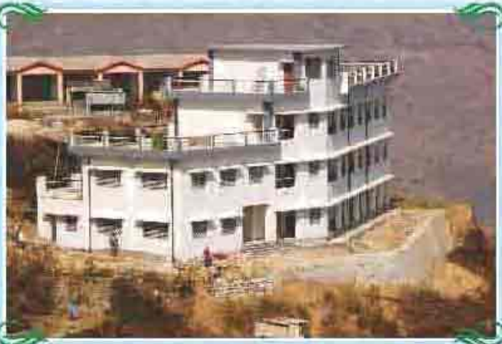
Building of Dr. Arbedkar SC/ST Hostel at New Thri
