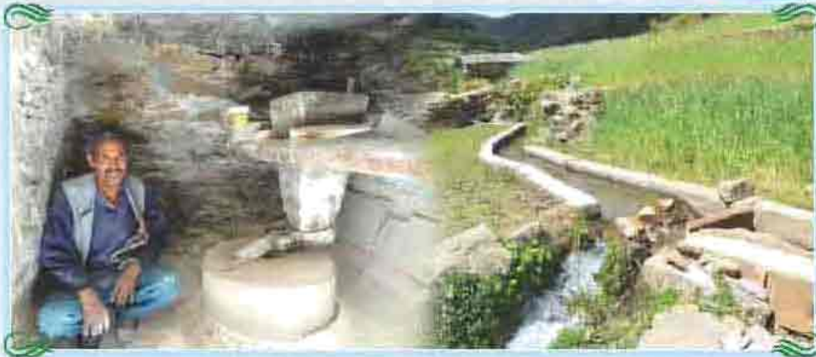
Restoration of Old Gharats (Panchakiri) at Deogagan Area, Distt. Tehri
