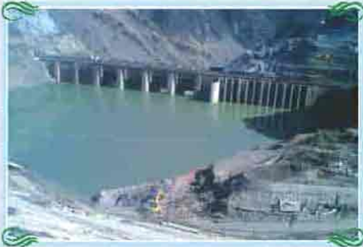
Up Stream view of Koteshwar Dam
