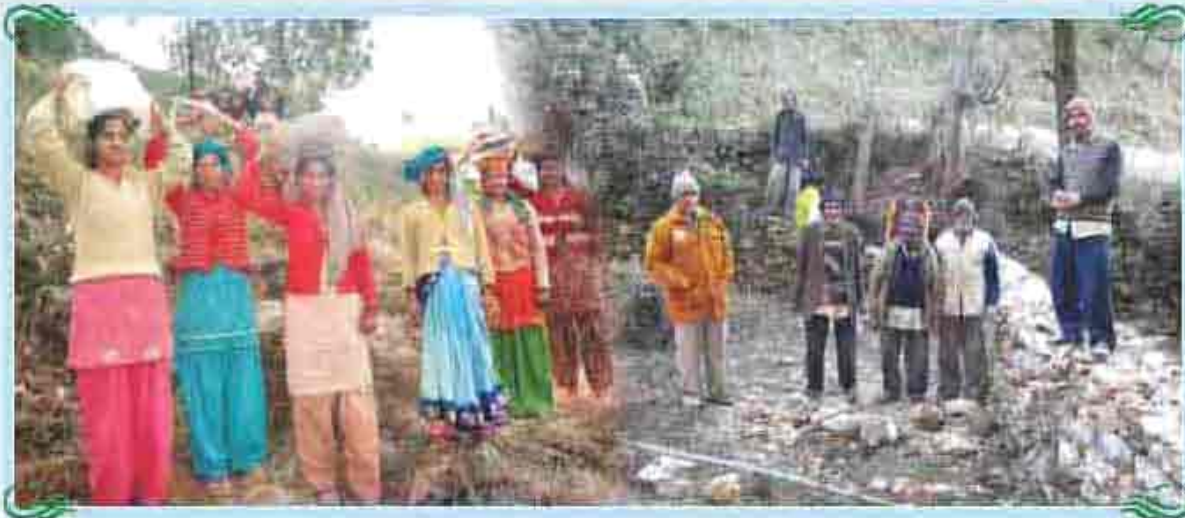
Slope Stabilisation work in the Tehri Dam Catchment Area
