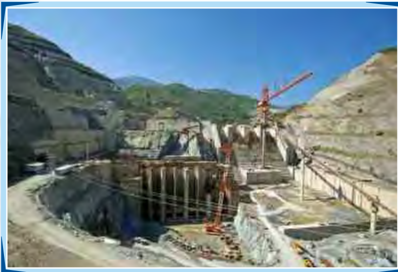
Work-in-Progress at Koteswar HEP (400 MW)
