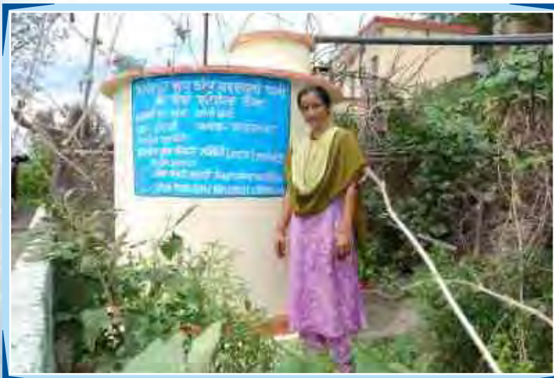
Rain water harvesting infrastructure set up by SEWA - THDC for the villagers in and around Tehri
