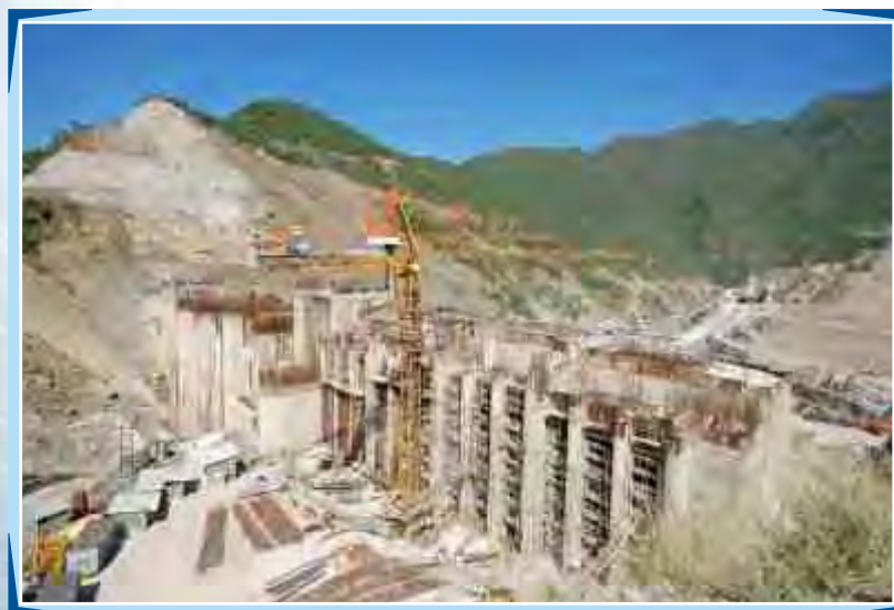
Work-in-Progress at Koteswar HEP (400 MW)
