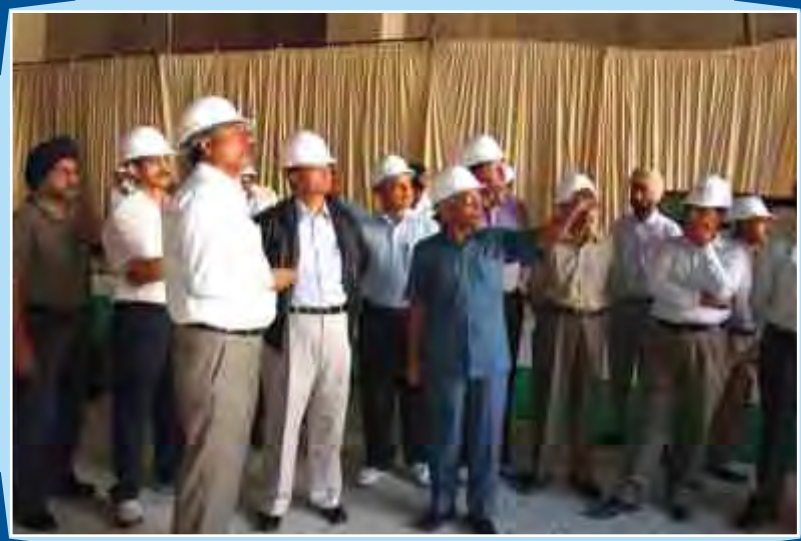
Shri Harishankar Brahma, Secretary (Power), inspecting the ongoing construction works at Koteswar HE Project.
