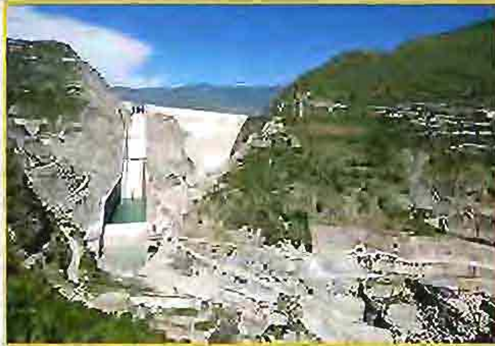
View of Asia's Highest Tehri Dam & Chest Spway
