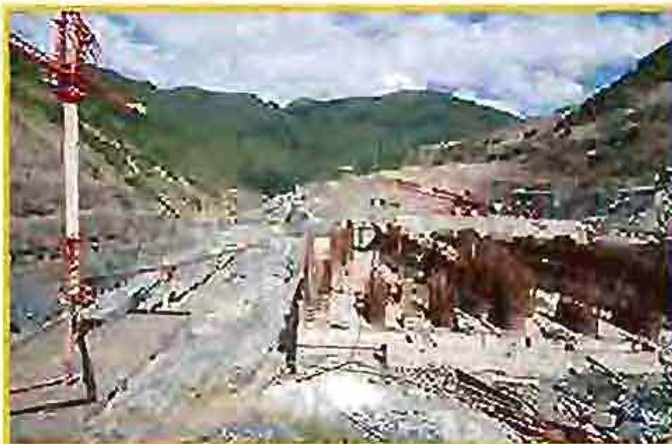
Work-In-Progress at Kozhaswar HE Project
